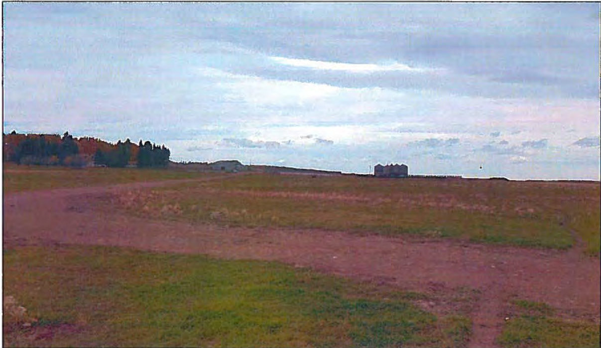
Photograph No. 1: Photograph taken from near Borehole BH103, facing northwest, showing the majority of the proposed feedlot expansion footprint, existing feedlot and associated infrastructure, site grading, and site conditions at the time of drilling. Photograph taken on the 30 th September, 2021.
