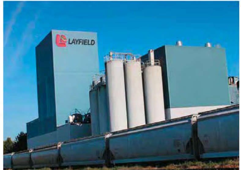
Figure 1. Layfield's headquarters and manufacturing facility in Vancouver, Canada.
