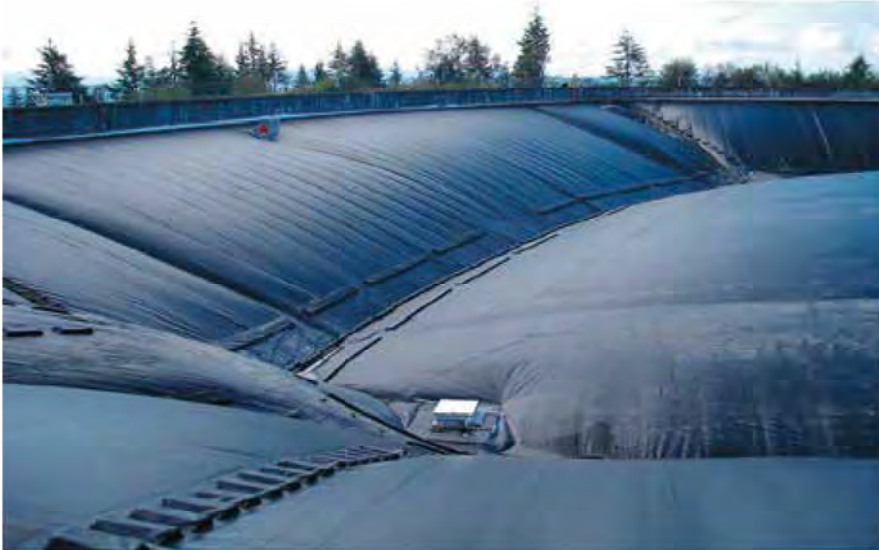
Figure 28. Floating cover being inflated during inspection
