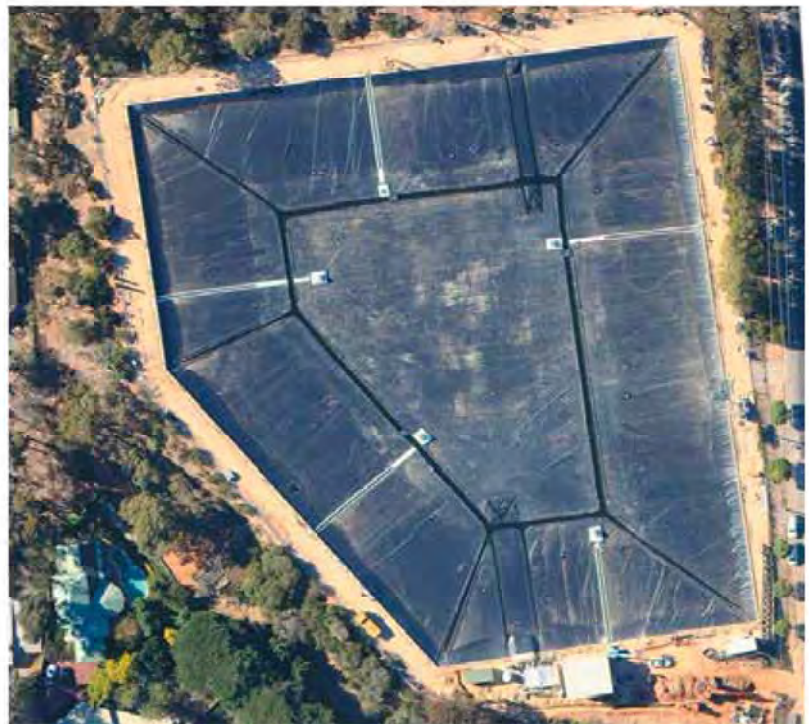
Figure 10. Enviro Liner® 6040 defined sump floating cover for a potable water reservoir in Australia
