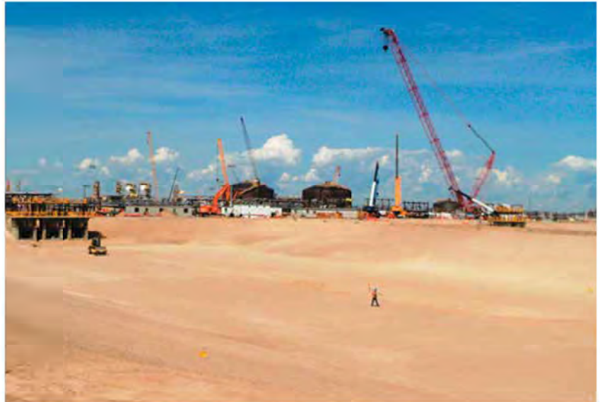
Figure 26. Approved subgrade for an oilsands project in Northern, Alberta
