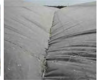
Figure 8b. Inflated Enviro Liner® 6030 Cap
