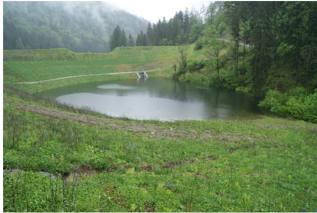
Figure 172-3 Test Storage to ~1/3 (10 m) of the Structure Height at Lankowitzbach
