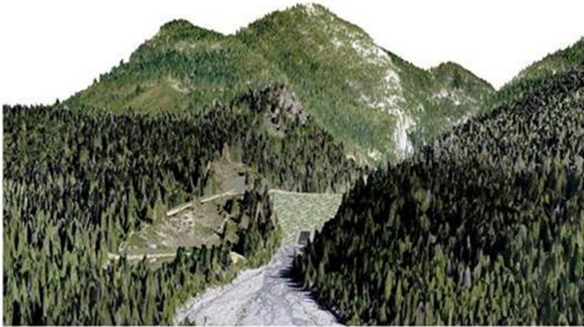
Original vegetated spillway design – no water impoundment
