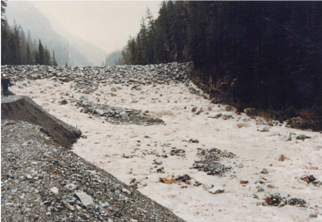
Photo 3-1. Upstream view of Cougar Creek Dam 1 hour before the failure. May 25, 1990 (Alberta Environment, 1991).
