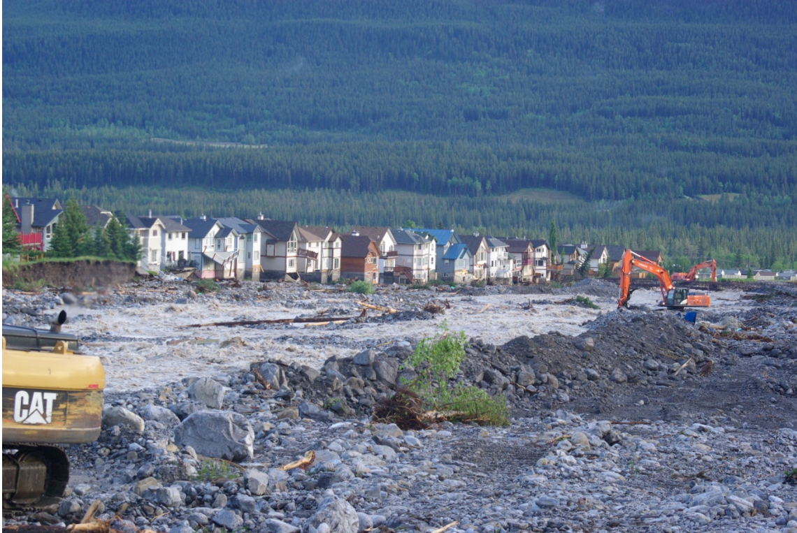
Photo A-21. Downstream view of Cougar Creek looking to homes on the left (east) bank along Grotto Road. Photograph courtesy of the Town of Canmore.
