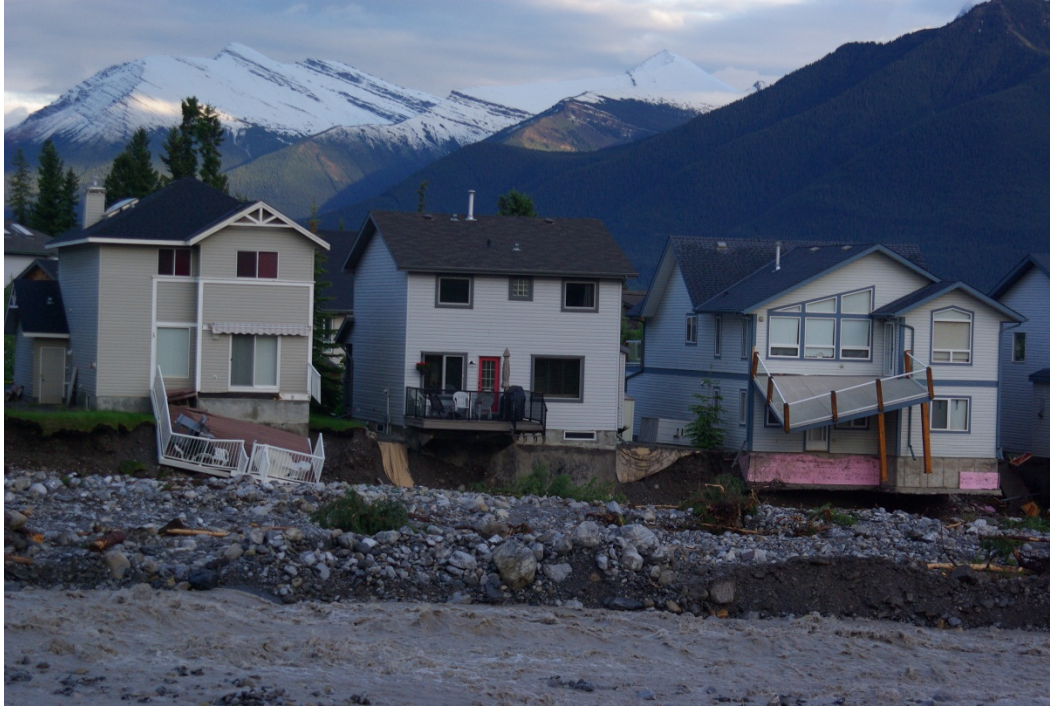
Photo A-25. Damage sustained to homes along the left (east) bank of Cougar Creek along Grotto Road. Photograph courtesy of the Town of Canmore.
