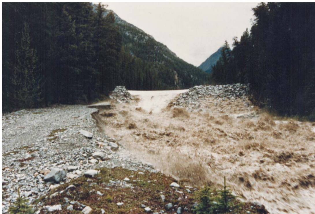
Photo 3-3. Upstream view of Cougar Creek Dam shortly after the breach initiated. May 25, 1990 (Alberta Environment, 1991).
