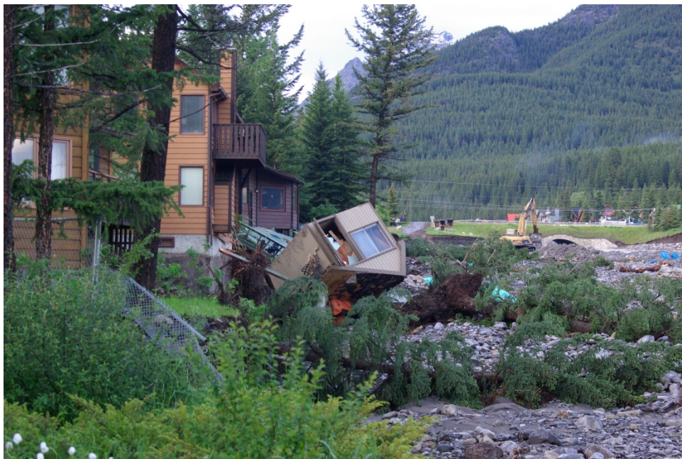
Photo A-22. Damage sustained to house along the right (west) bank of Cougar Creek along Coyote Way. Photograph courtesy of the Town of Canmore.
