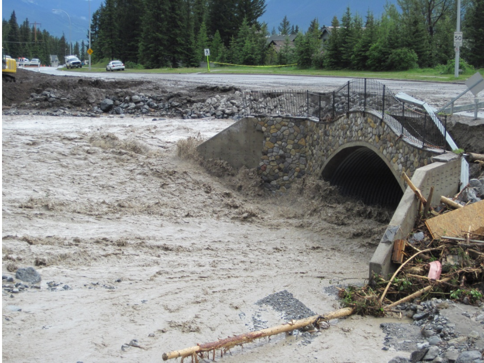
Photo A-5. Side view of inlet to Elk Run Boulevard culvert. Note the outflanking of the culvert that has occurred. Photograph courtesy of the Town of Canmore.
