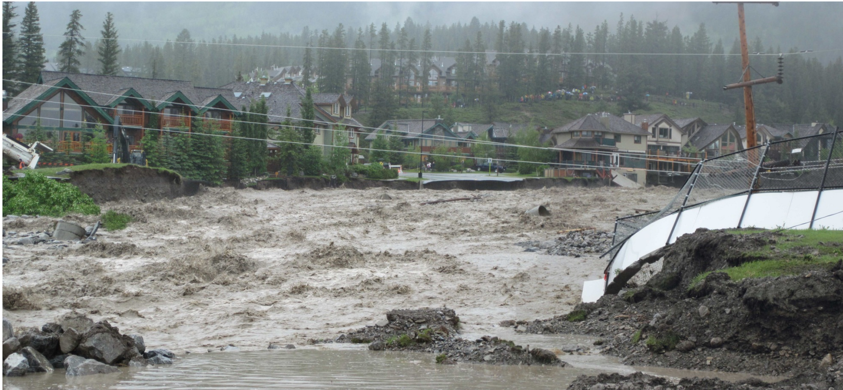
Photo A-7. Upstream view of Cougar Creek from Elk Run looking over to the right bank and the eroded Benchlands Trail. A severely damaged outdoor hockey rink is visible in the foreground. Photograph courtesy of the Town of Canmore.
