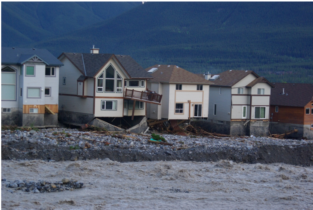
Photo A-24. Damage sustained to homes along the left (east) bank of Cougar Creek along Grotto Road. Photograph courtesy of the Town of Canmore.
