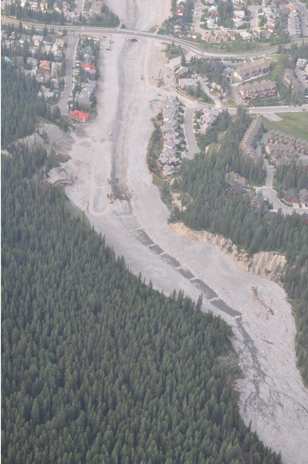
Photo A-38. Aerial view of reconstructed Cougar Creek looking downstream from about the fan apex. BGC photograph of July 23, 2013.
