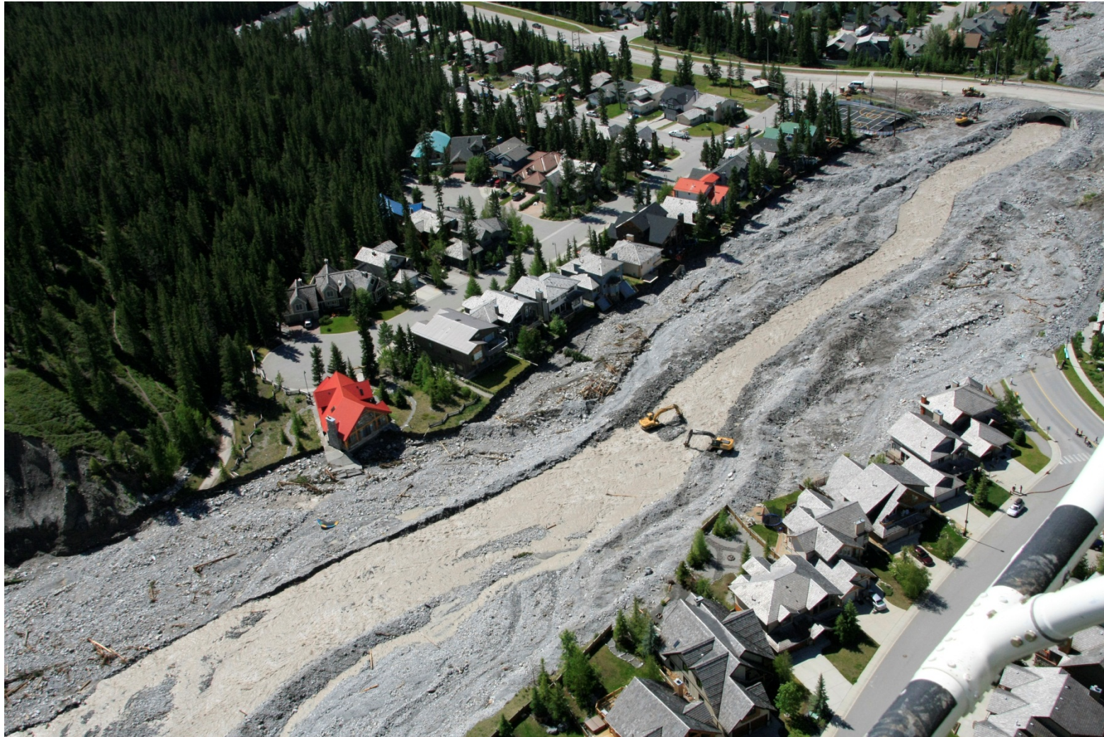
Photo A-11. Aerial view of restoration efforts along Cougar Creek upstream of Elk Run Boulevard following the 2013 debris flood. Photograph courtesy of the Town of Canmore.
