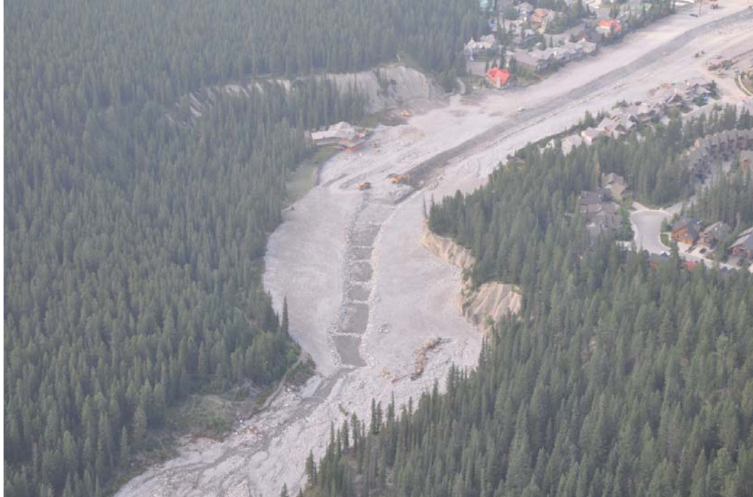
Photo A-40. Aerial view of reconstructed Cougar Creek looking downstream from about the fan apex. BGC photograph of July 23, 2013.
