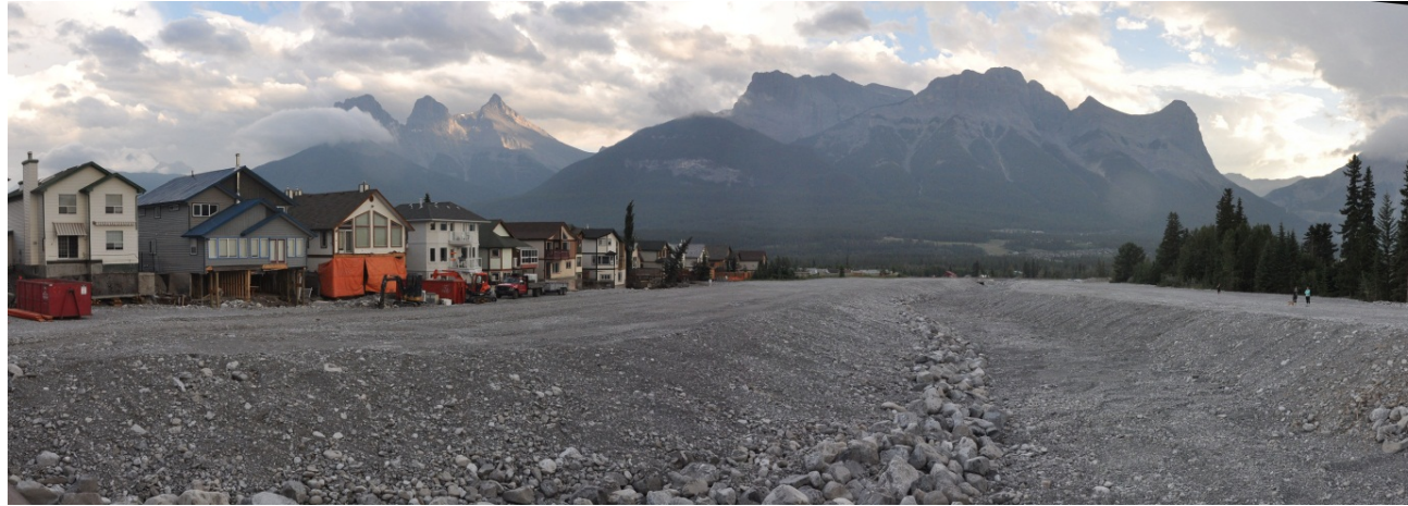
Photo A-35. Downstream view of reconstructed Cougar Creek channel from the pedestrian bridge. BGC photograph of July 23, 2013.
