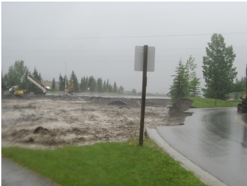
Photo A-6. Downstream view to Elk Run Boulevard culvert from Benchlands Trail, which has partially eroded. Photograph courtesy of the Town of Canmore.
