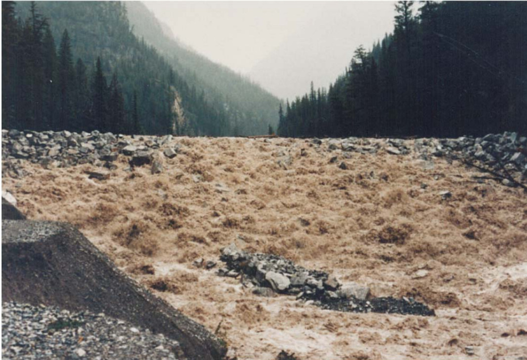
Photo 3-2. Upstream view of Cougar Creek Dam 10 minutes before the failure. May 25, 1990 (Alberta Environment, 1991).
