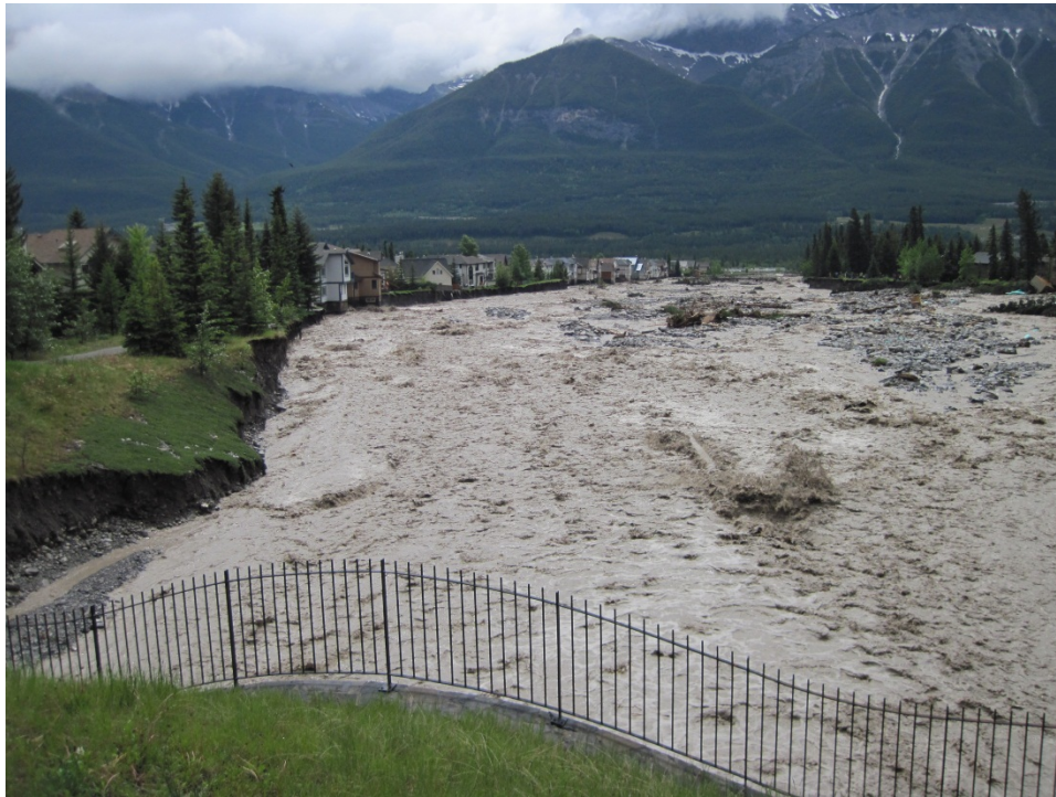
Photo A-15. Downstream view of Cougar Creek from Elk Run Boulevard. Note the left bank erosion adjacent to Lady Macdonald Crescent. Photograph courtesy of the Town of Canmore.
