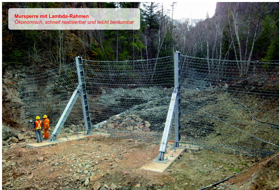
Photo 8-2. Debris flow net barrier with lambda-shaped frames and the possibility for structure opening for debris clearing in the centre of the structure
