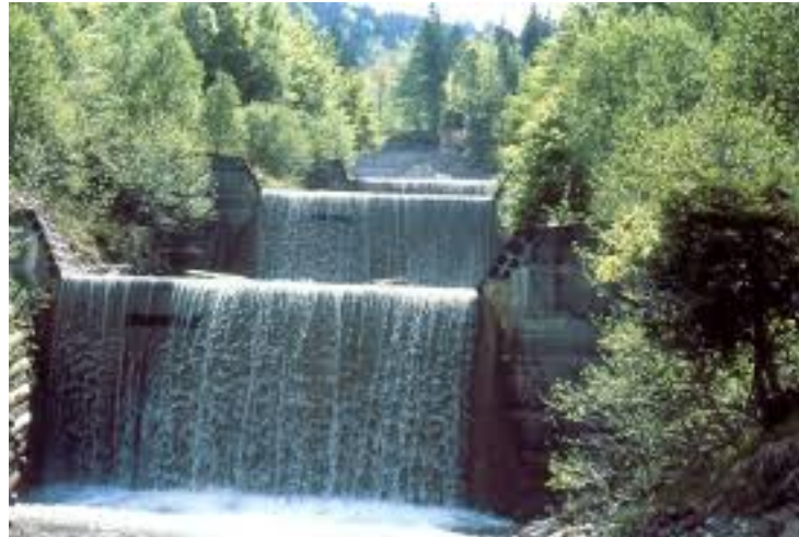
Photo 8-3. Example of a series of stepped concrete check dams. Location unknown.
