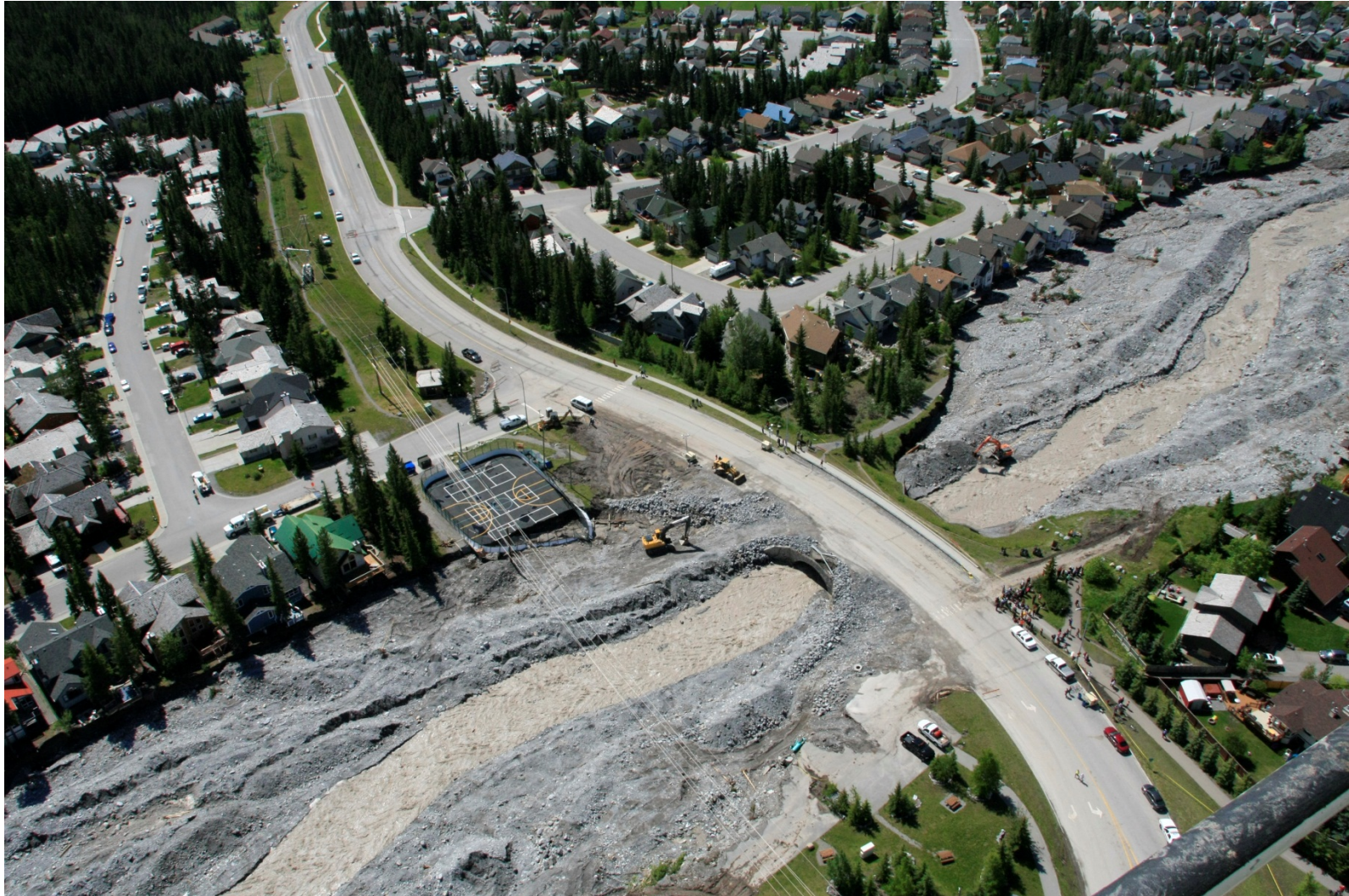
Photo A-12. Aerial view of restoration efforts along Cougar Creek at Elk Run Boulevard following the 2013 debris flood. Photograph courtesy of the Town of Canmore.
