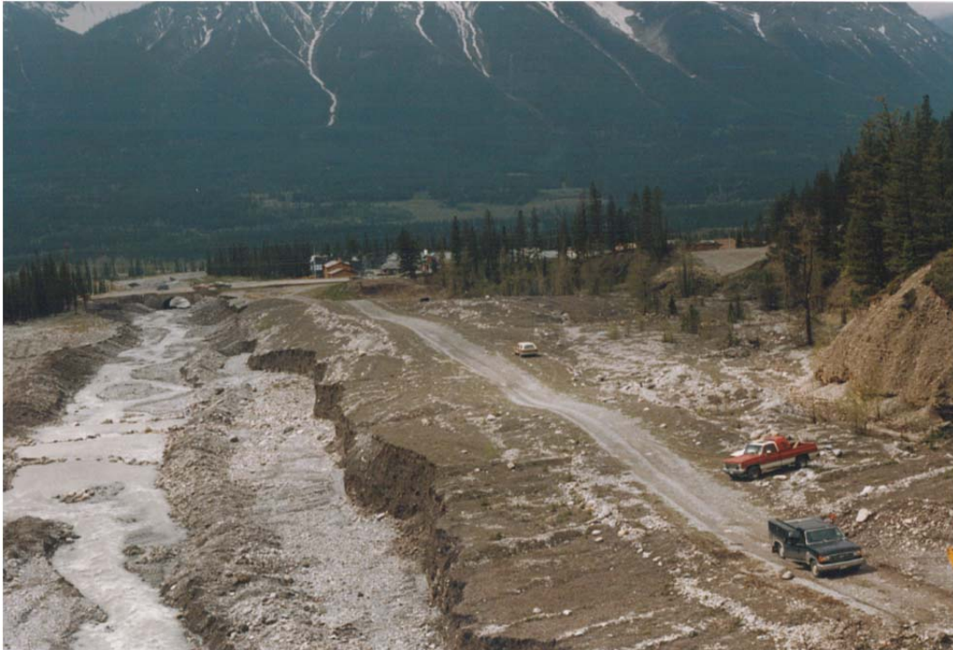
Photo 3-6. Downstream view of Cougar Creek looking toward Elk Run Boulevard. Photo courtesy of Kent Berg, Alberta Environment and Sustainable Resource Development. May 26, 1990.
