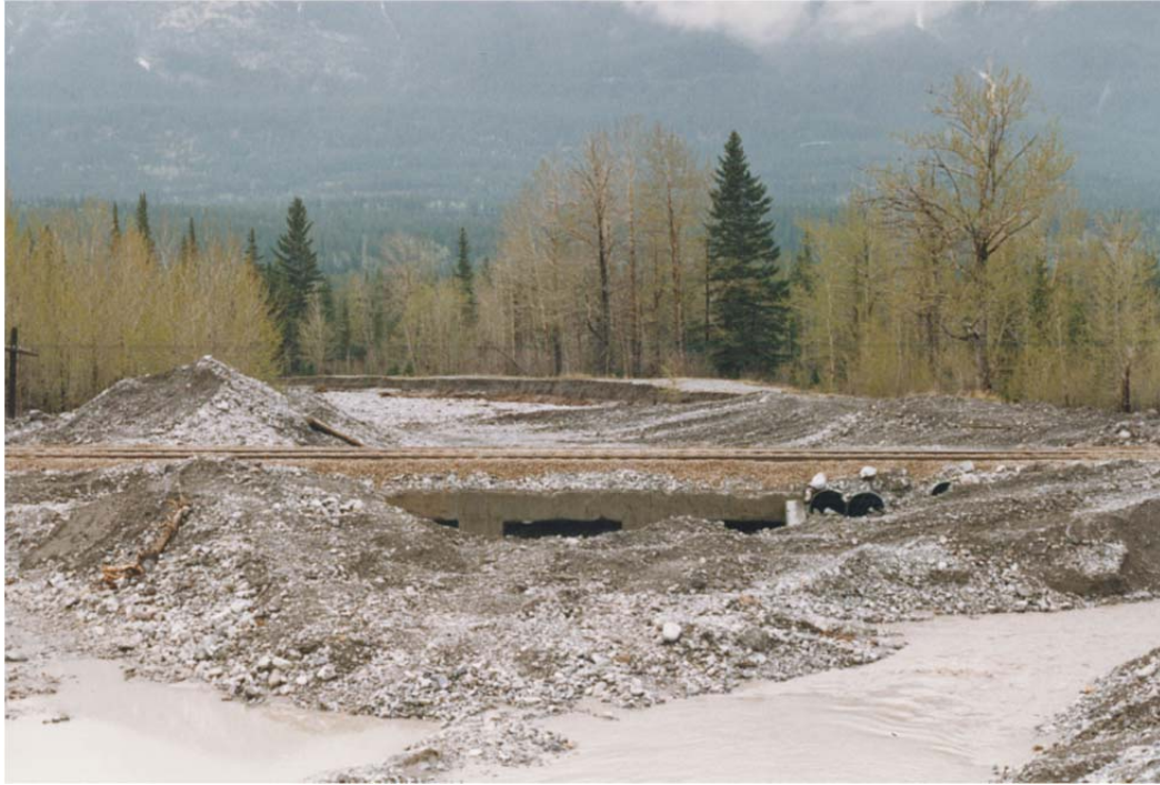
Photo 3-7. Aggradation at the CP Railway following the 1990 dam failure. Photo courtesy of Kent Berg, Alberta Environment and Sustainable Resource Development. May 26, 1990.
