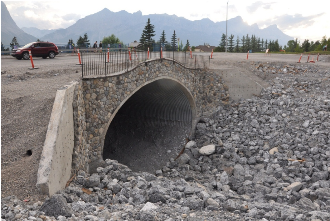
Photo 2-1. Culvert inlet at Elk Run Boulevard. BGC photograph of July 23, 2013.
