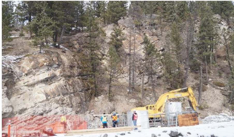
Figure 11: Rock outcrop at the right abutment (Photo: ALPINFRA 2014)
