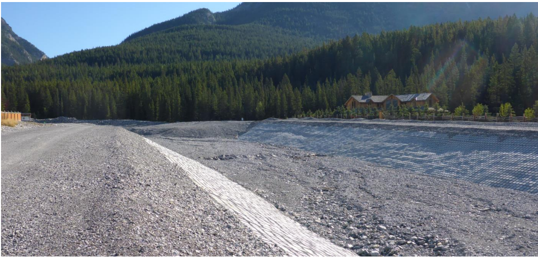
Figure 6: Reinforced downstream channel
