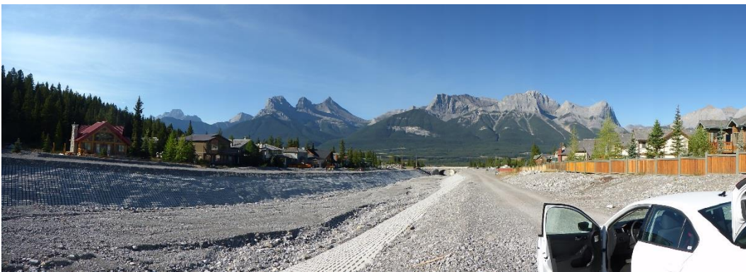
Figure 7: Downstream channel and culvert of Bow Valley Trail with houses next to Cougar Creek channel
