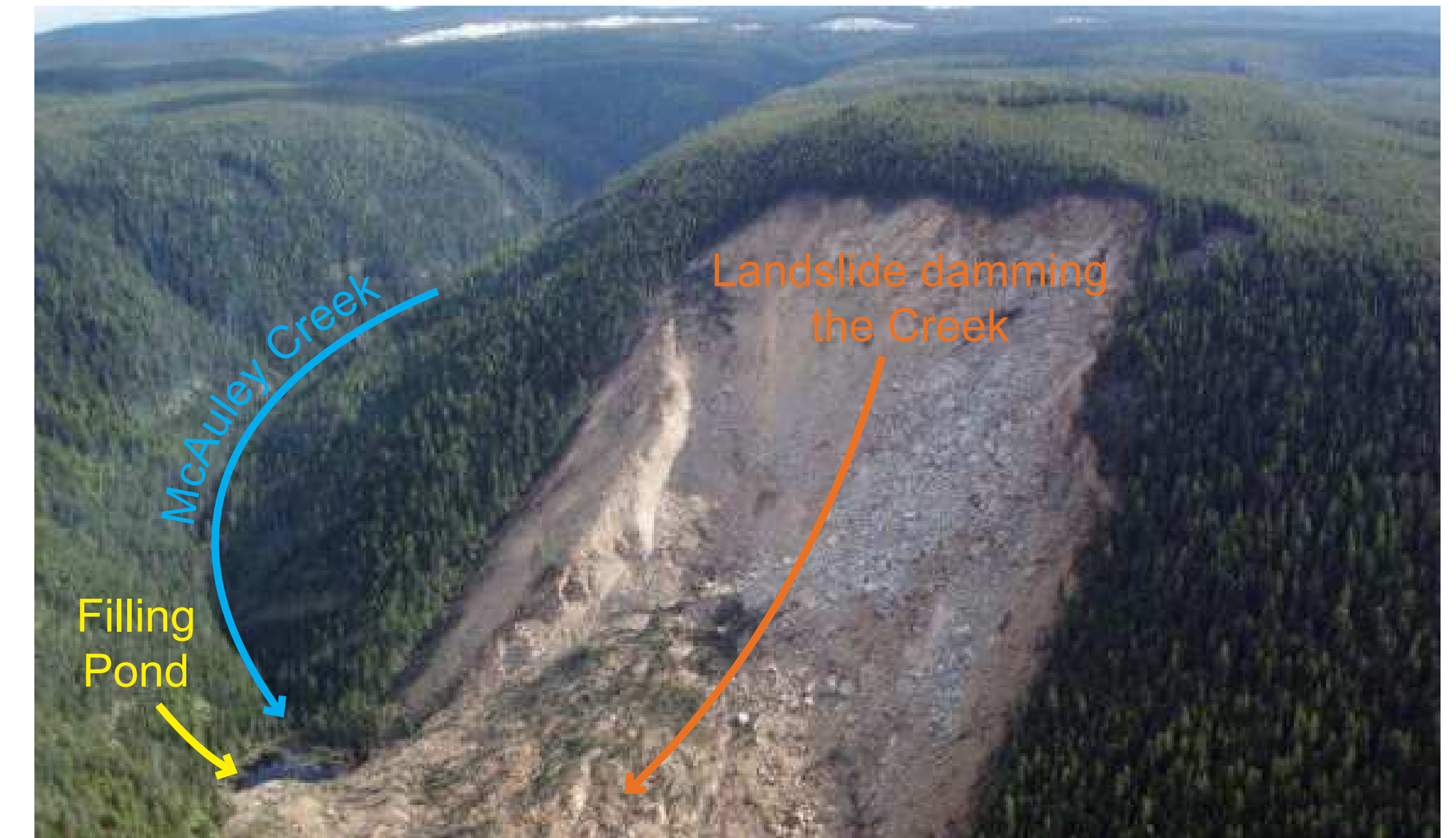
Landslide Dam Outbreak Flood at McAuley Creek Slide near Vernon, BC
