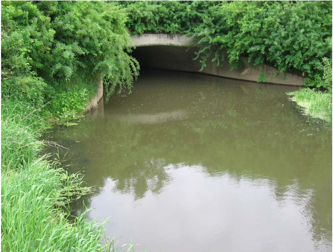
Photo III-10: Surface Water Monitoring Location BC-DS looking East (June 14, 2006)
