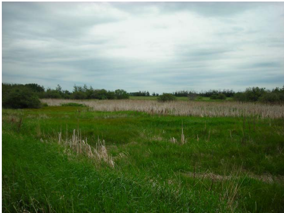
Photo I-8: Southeasterly View of Dugout in Wetland 01 with Power Substation in Background (June 2006)
