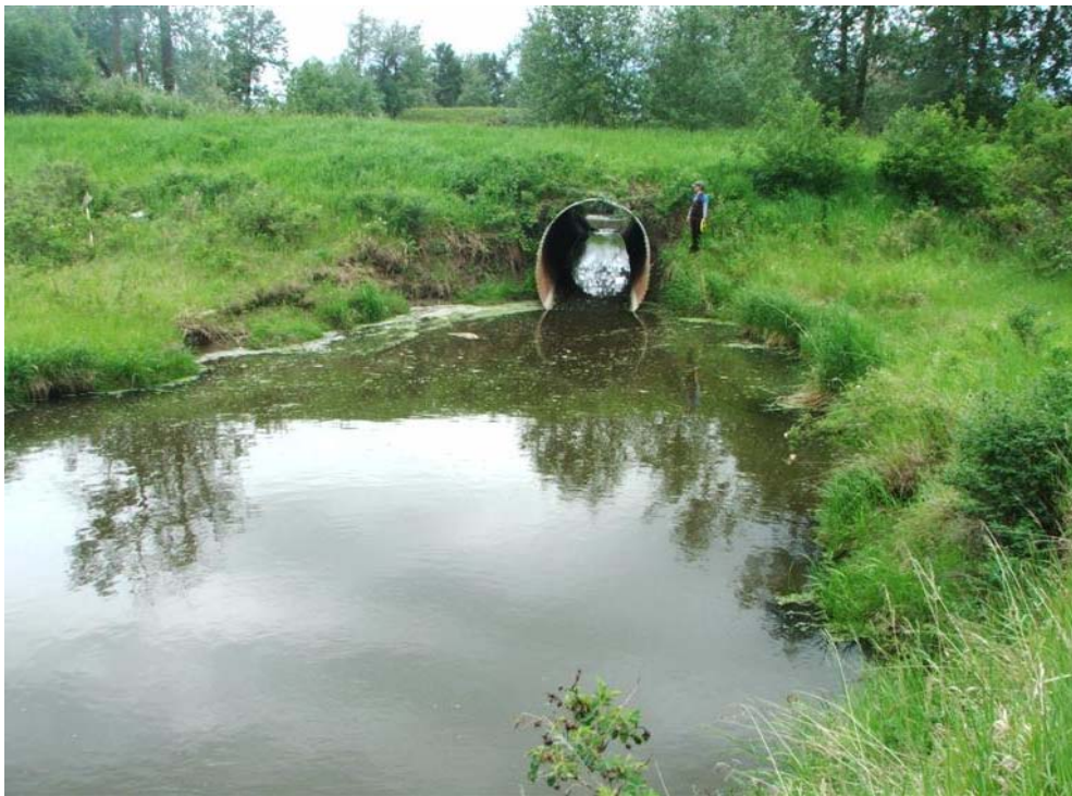
Photo I-10: Upstream View of Lamont Creek and Culvert Under Twp Rd 560 (June 2006)
