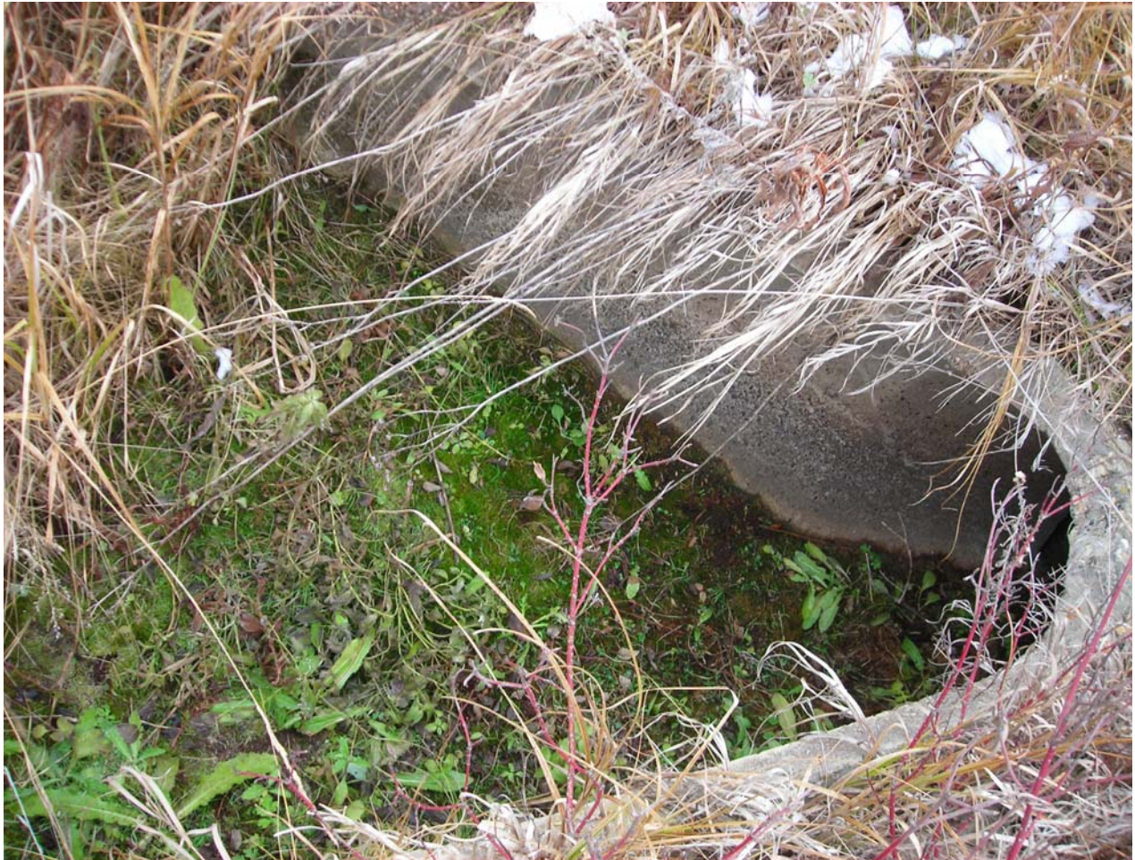
Photo III-8: Sediment Sampling Location SED8 (October 18, 2006). No Free Water, only Sediment was Sampled at this Location. Conveyance under Highway 45 is via two 760 mm Concrete Pipes mitred to Bank
