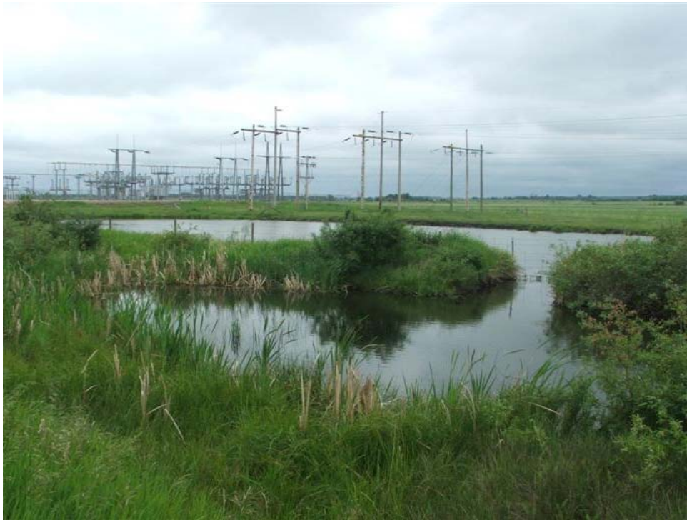
Photo I-5: Southeasterly View of Dugout in Wetland 01 with Power Substation in Background (June 2006)
