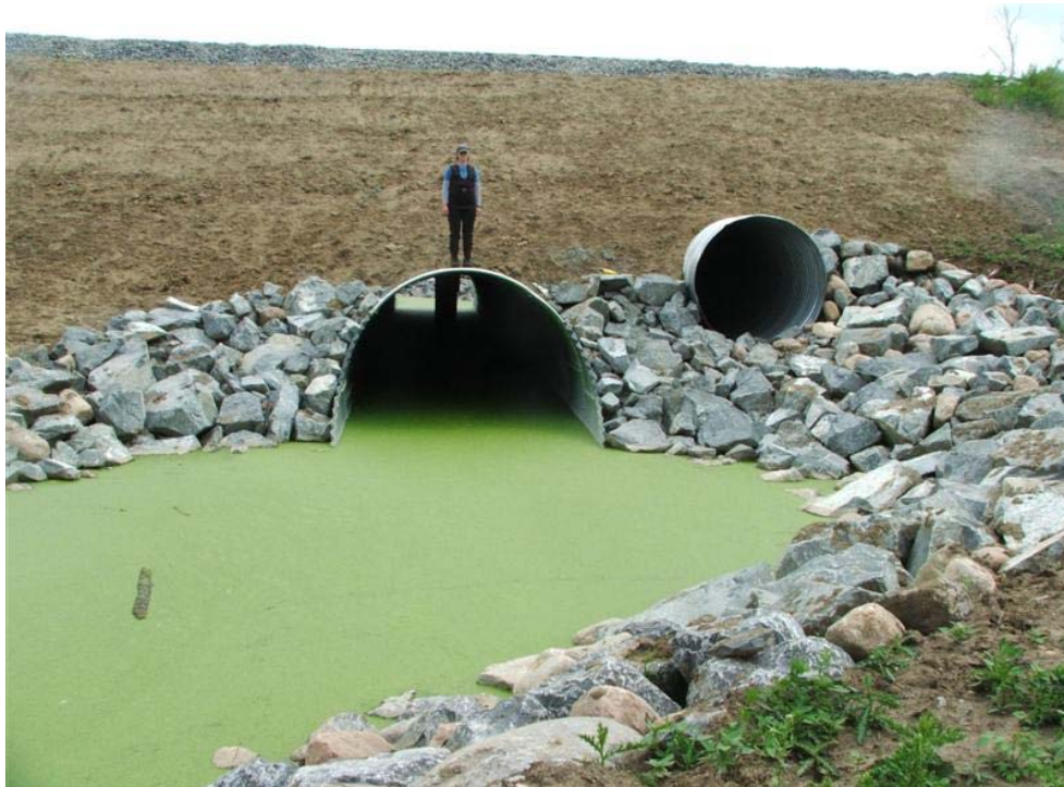
Photo I-13: Upstream View of Culvert at Railway Crossing of Lamont Creek (June 2006)
