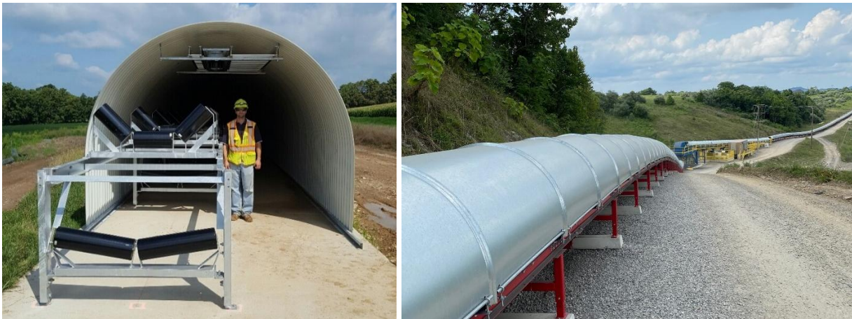
Examples of shrouded overland conveyors. The 4.5 km conveyor proposed as part of the Scott Project will eliminate greenhouse gas emissions and public safety concerns associated with aggregate haul traffic.
