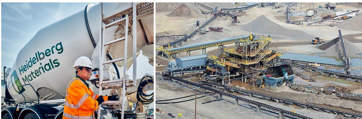
Heidelberg's Spy Hill facility includes aggregate processing equipment, a ready-mix concrete plant, and a concrete pipe manufacturing plant. Heidelberg has invested in new technologies at this facility to increase energy efficiency and improve water management, leading to greenhouse gas reductions and improved water conservation.
