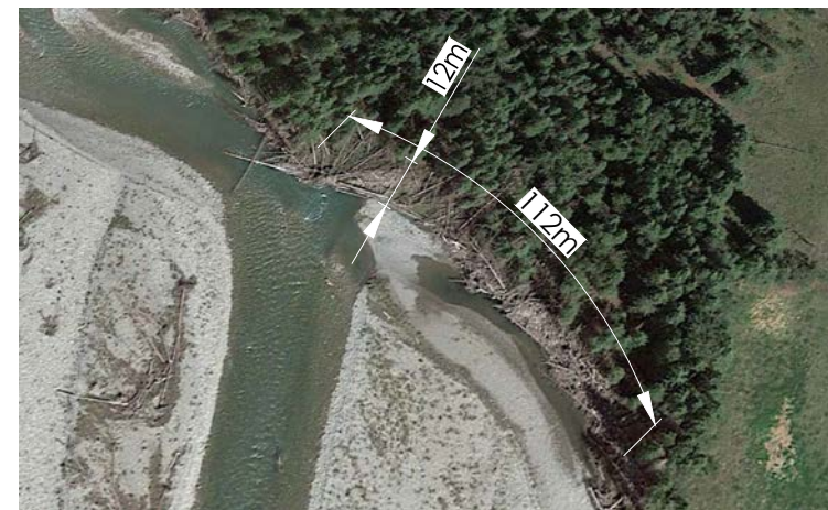
D DEBRIS JAM ALONG RIVER BANK (DEBRIS JAM DIMENSIONED)
