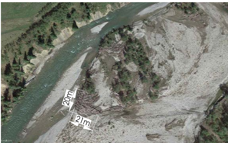
A DEBRIS JAM AT NOSE OF A BENCH (DEBRIS JAM DIMENSIONED)
