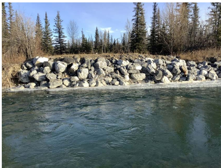
Photo A-16 Fall 2019 Photo of Elbow River Armoured Bank Lateral Scour Pool Macrohabitat Unit
