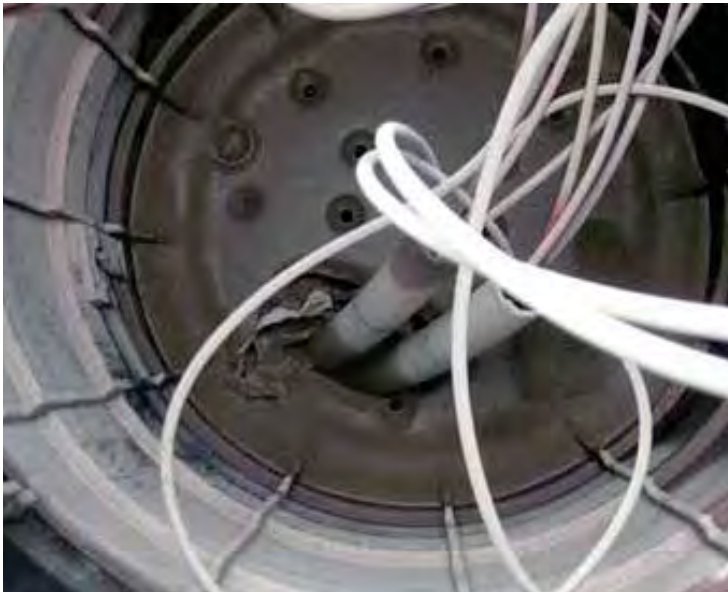
Fig. 13 - In Grade JB - Mud accumulation
