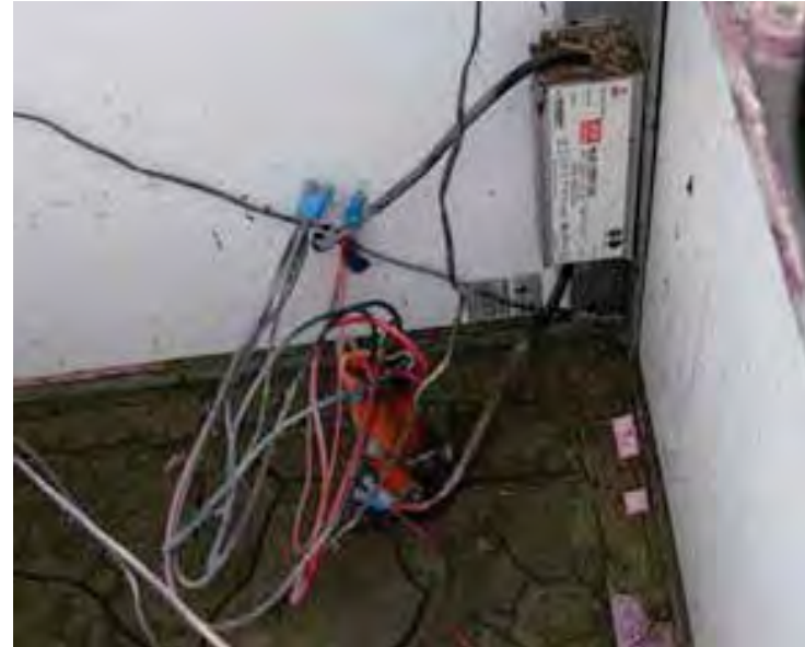
Fig. 8 - Cube Driver - Fully submerged with condensation build up
