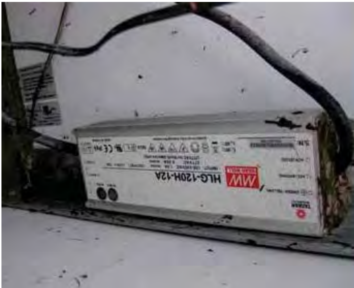
Fig. 9 - Cube Driver - Fully submerged
