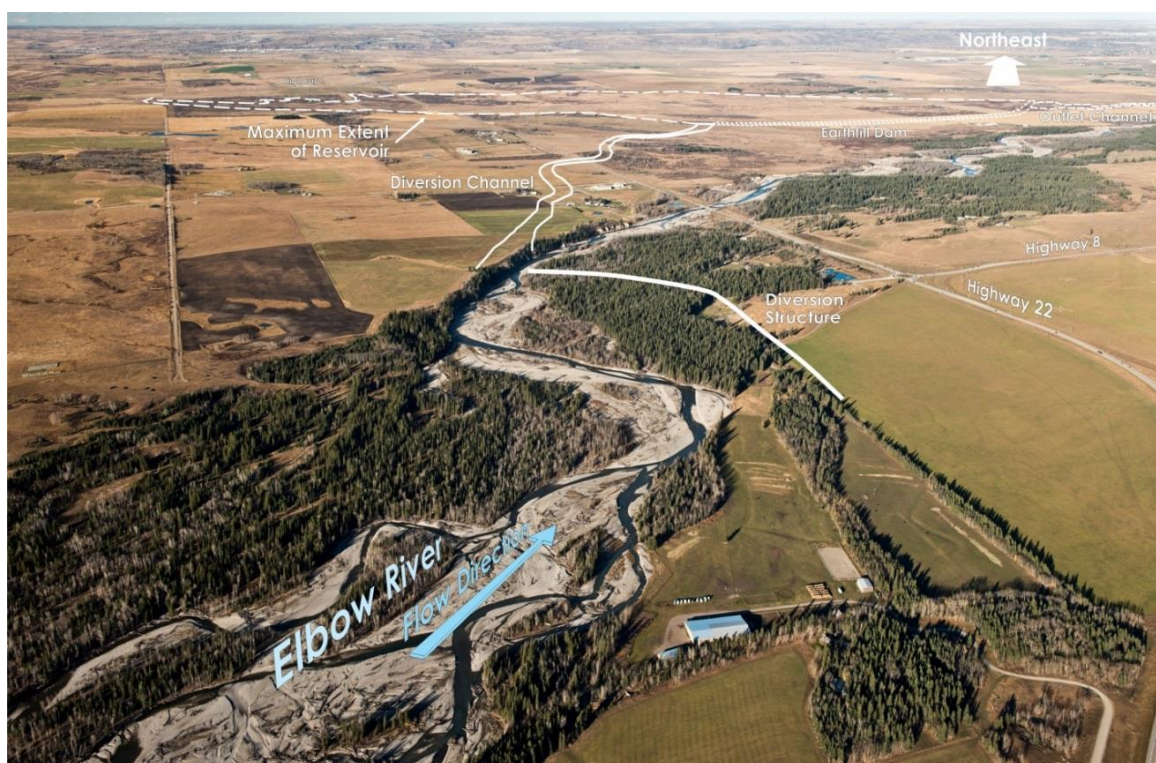
Figure 3. Looking Northeast towards Diversion Structure and Diversion Channel
