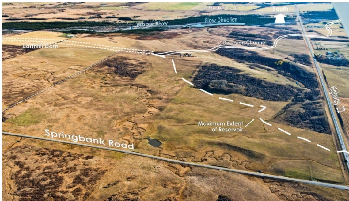
Figure 2. Looking South towards the Reservoir, Dam and Diversion Channel
