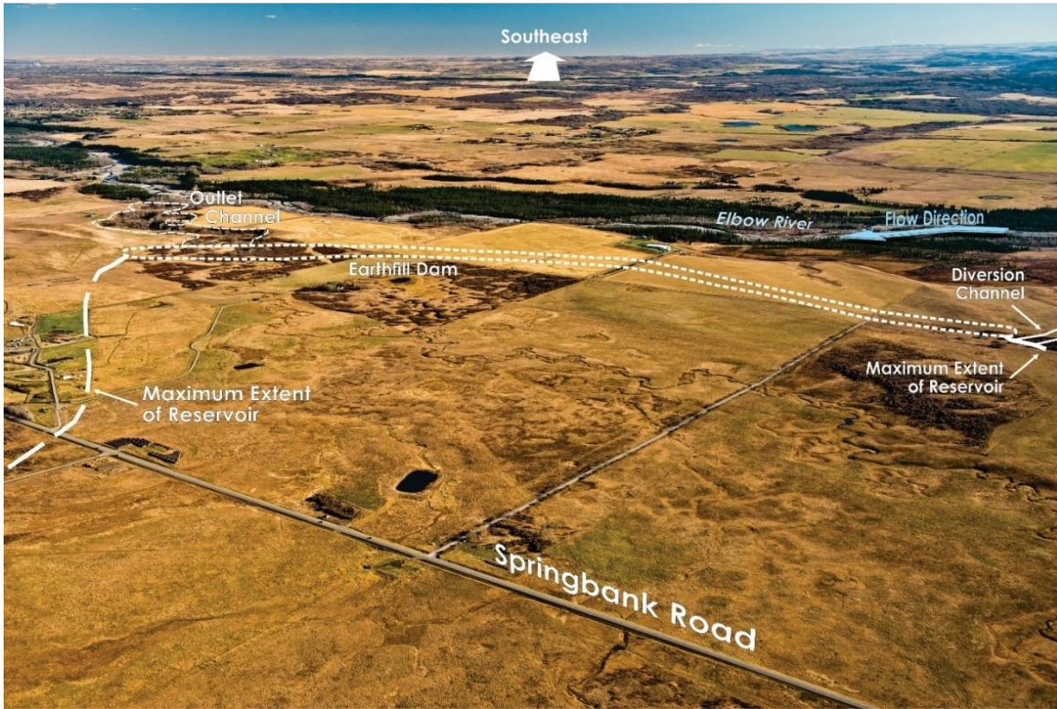
Figure 1. Looking Southeast towards Off-Stream Storage Reservoir and Dam
