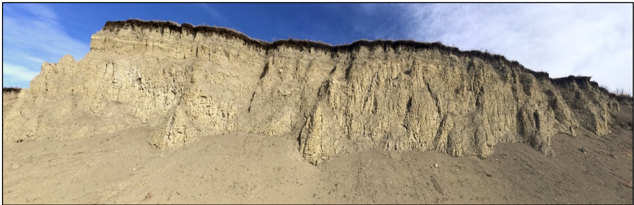
Figure 23. Rhythmically-bedded Glacio-lacustrine clay and silt observed in the upper part of OC14.
