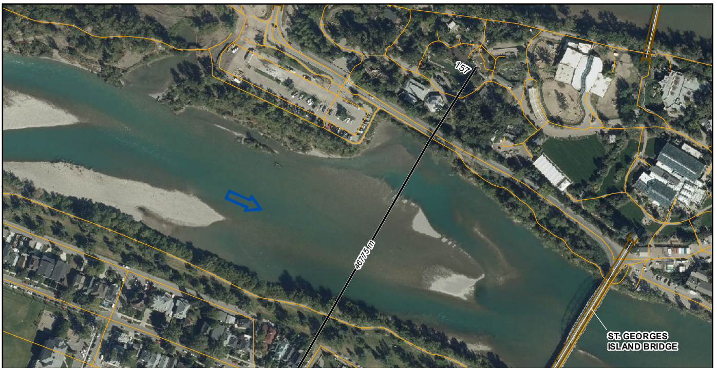
(2) AFTER THE 2013 FLOOD
