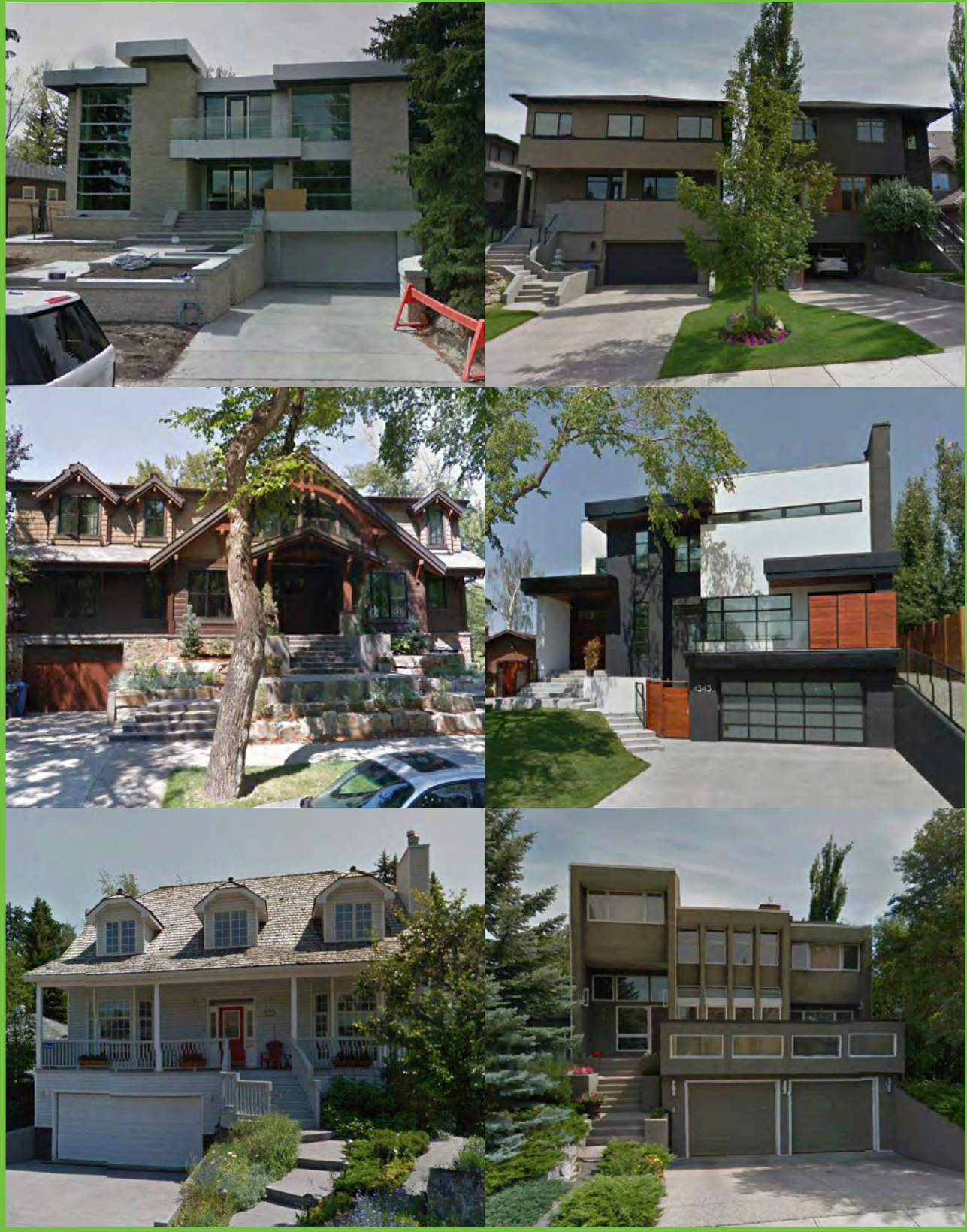
Single family homes with elevated main floor
