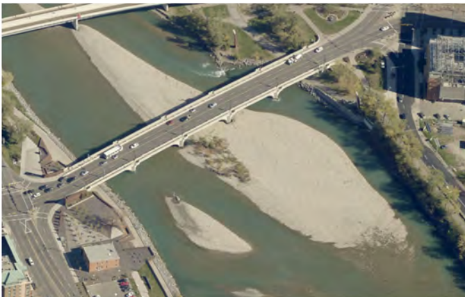
Gravel deposition at the Hillhurst-Louise Bridge
