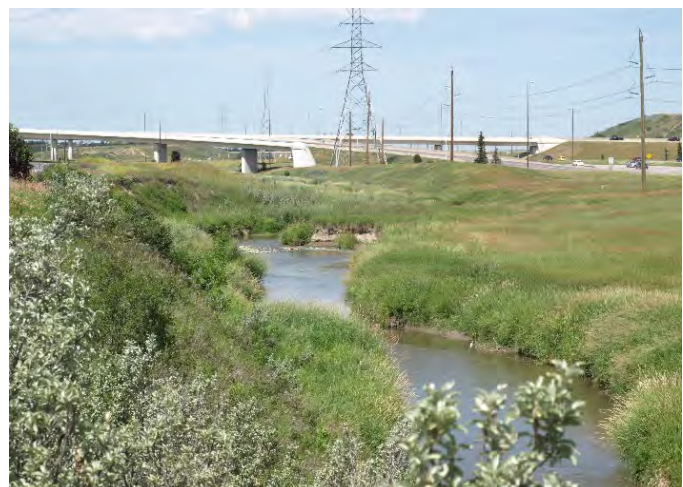
Realigned reach of Nose Creek
