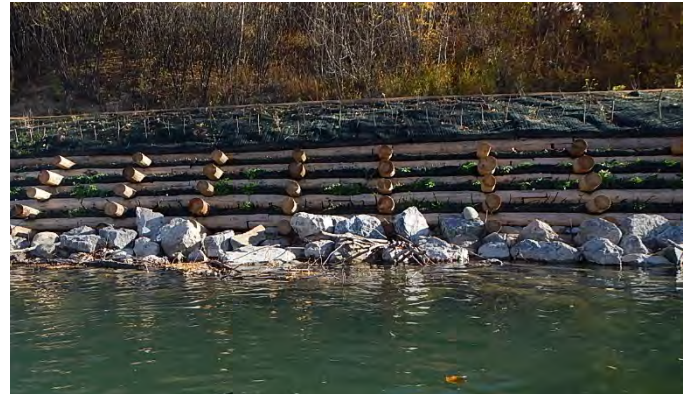
Timber crib wall with riprap toe on the Elbow River
