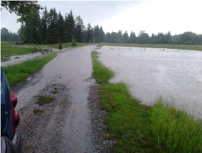
Looking east, the road leading into our main house yard, Flood, June 2013.
