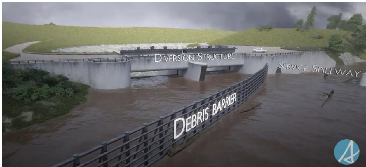
Figure 2. Schematic of Diversion Inlet, Debris Barrier, and Service Spillway along Elbow River, looking north (Source: Government of Alberta)
