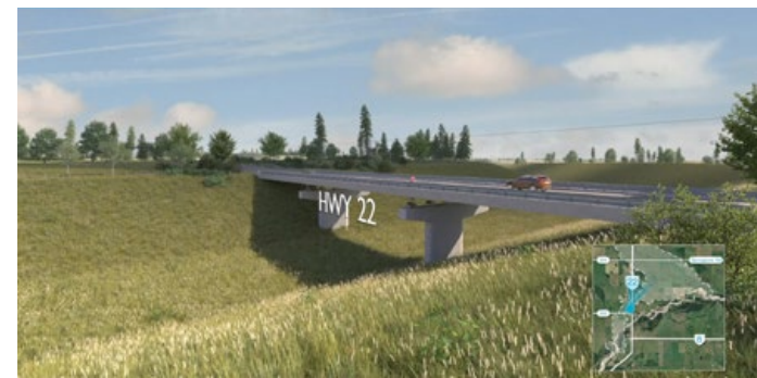
Highway 22 Bridge over the diversion channel during normal conditions
