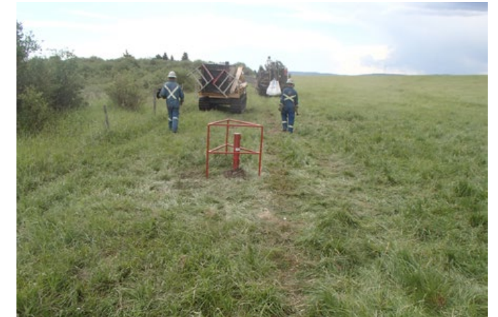
Example of a single monitoring well installation
