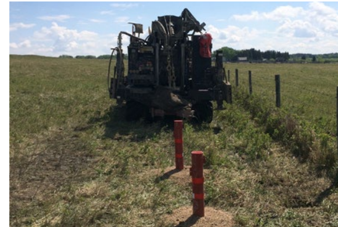
Example of a nested monitoring well installation for monitoring of groundwater at multiple depths
