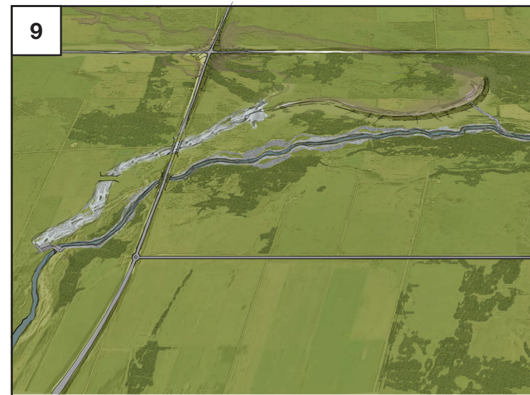
9 Once the reservoir has emptied back into the Elbow River, AEP operations and maintenance staff clear the channel of any problematic sediment or debris (if any).
