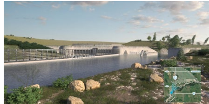
Diversion structure and service spillway gates during normal conditions
