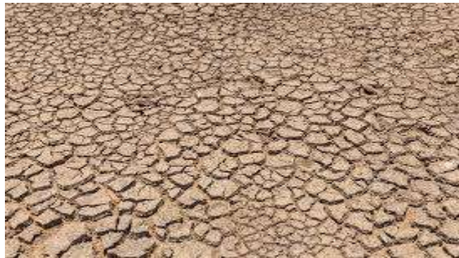
Ground cracking and increased seepage risk
