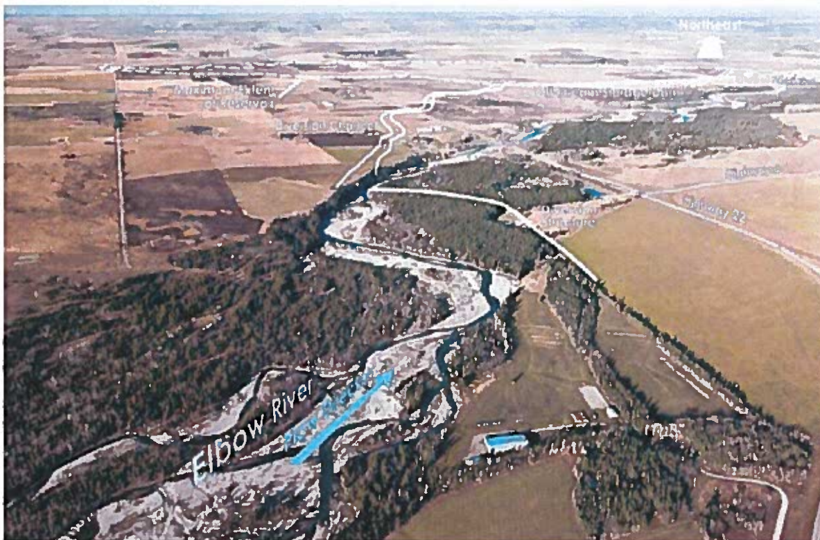
Figure 3-4 Looking Northeast towards Diversion Structure, Diversion Channel, Off-stream Storage Reservoir and Off-stream Storage Dam Locations
