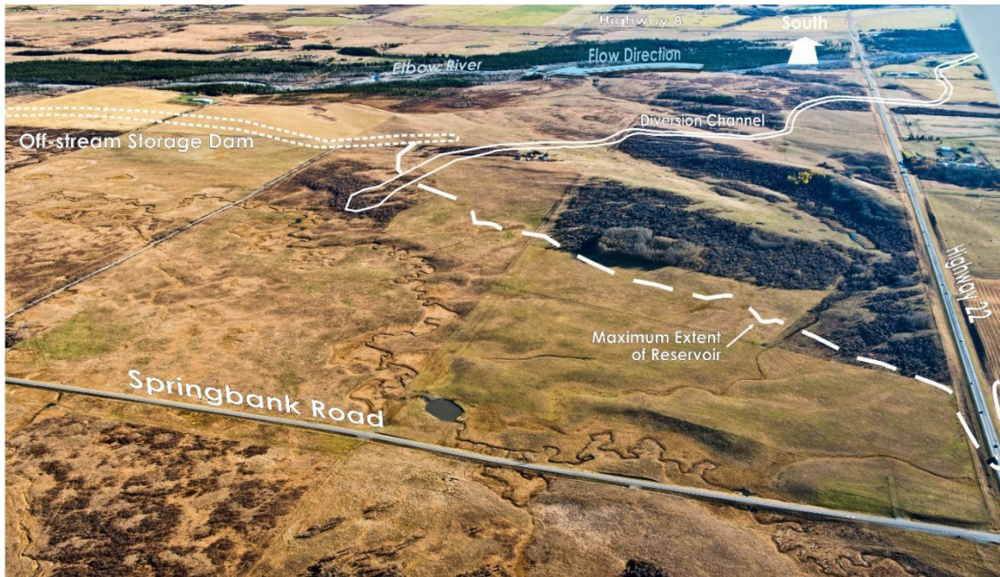
Figure 1-3 Looking South towards the Reservoir, Dam and Diversion Channel
