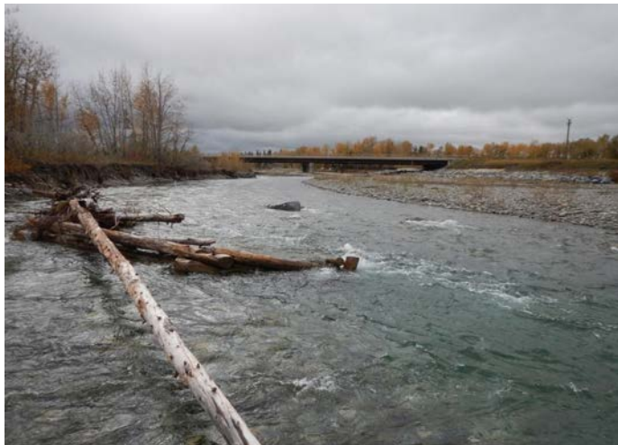
Photo 1: Looking upstream from T1 at the Highway 22 Bridge.
