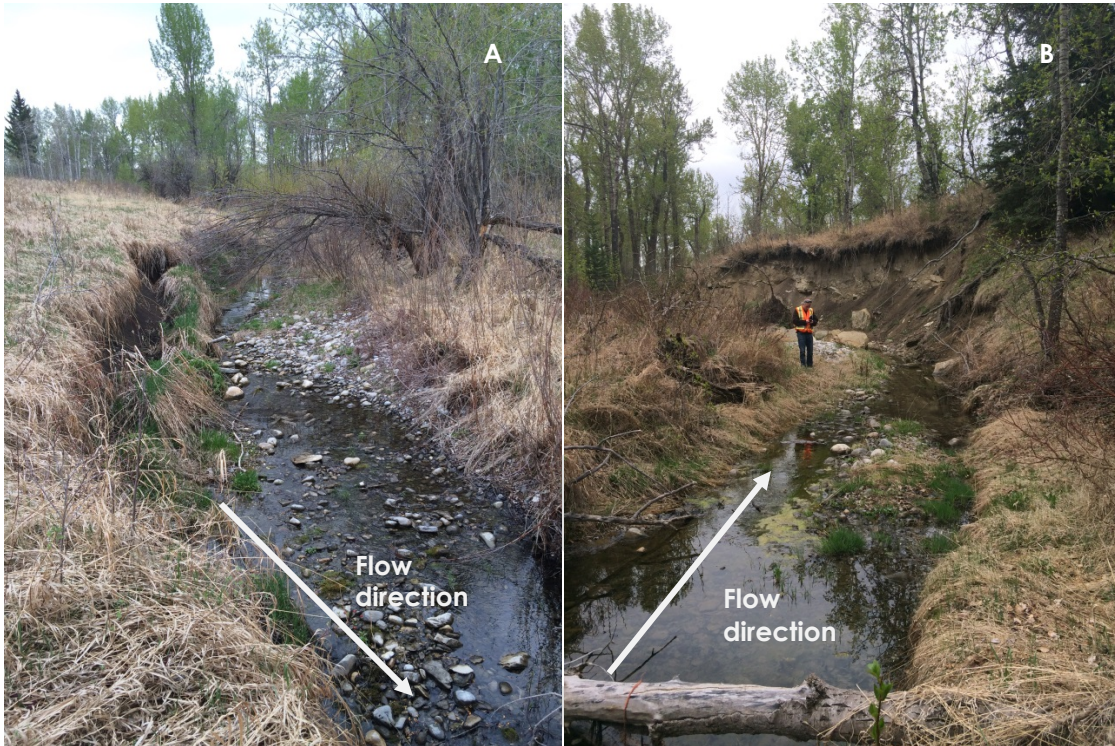
Figure 2-1 Outlet Channel – note bank collapse induced by toe cutting on true right bank. Locations of A and B are show in Figure 4-1
