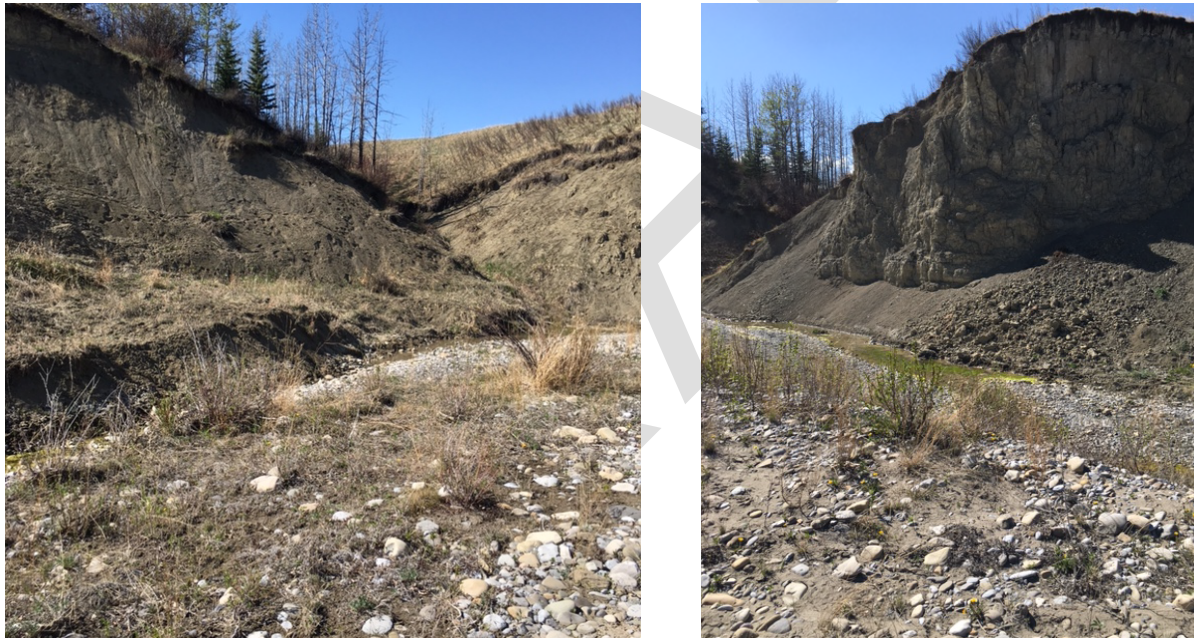
Figure 1. West Gully (left) and East Gully (right).
