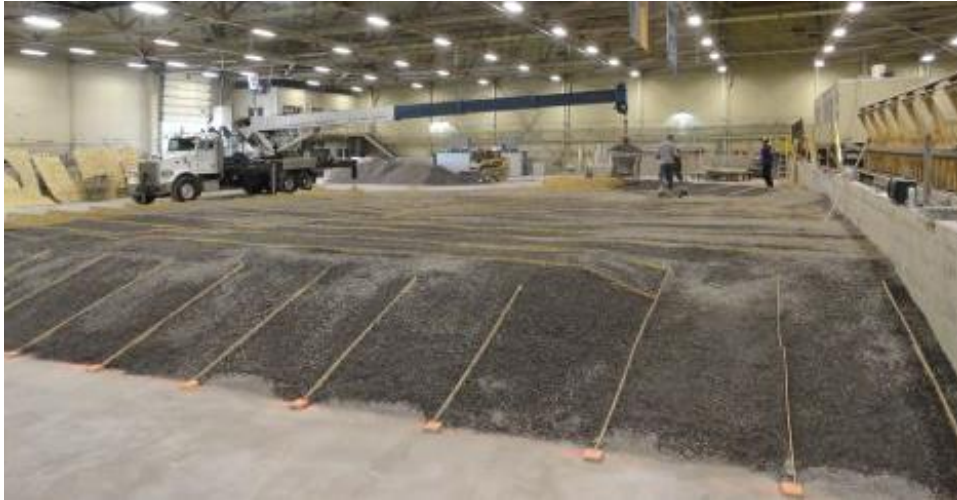
Figure 29. Heavy construction equipment was used to pour concrete.
