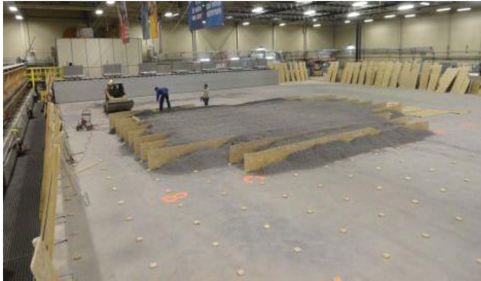
Figure 27. Fibreboard templates were erected and backfilled with fine gravel.
