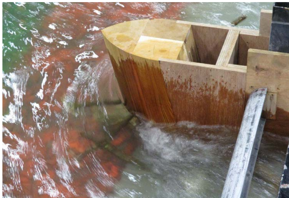
Figure 145. Debris caught on Pier Nose 3.
