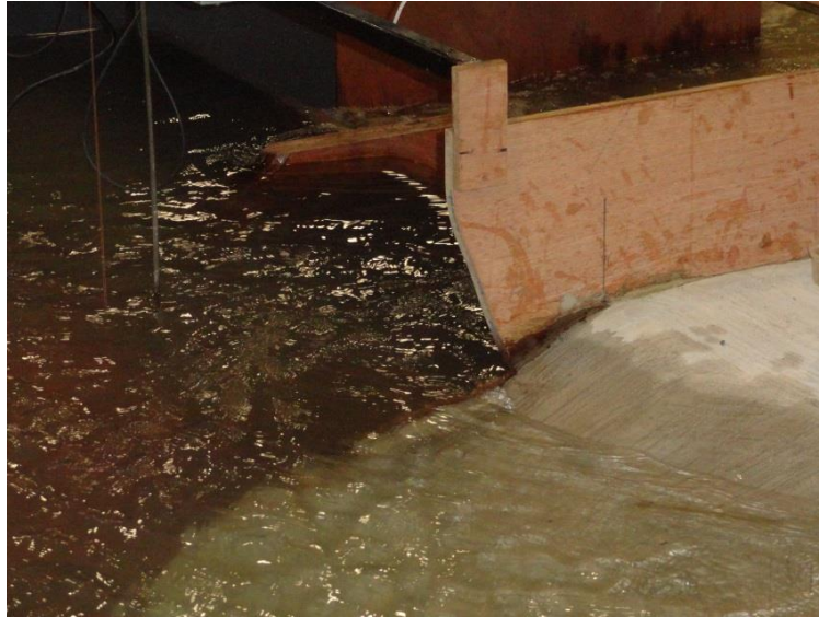
Figure 110. Cut-out section of retaining wall at RHS of service spillway.
