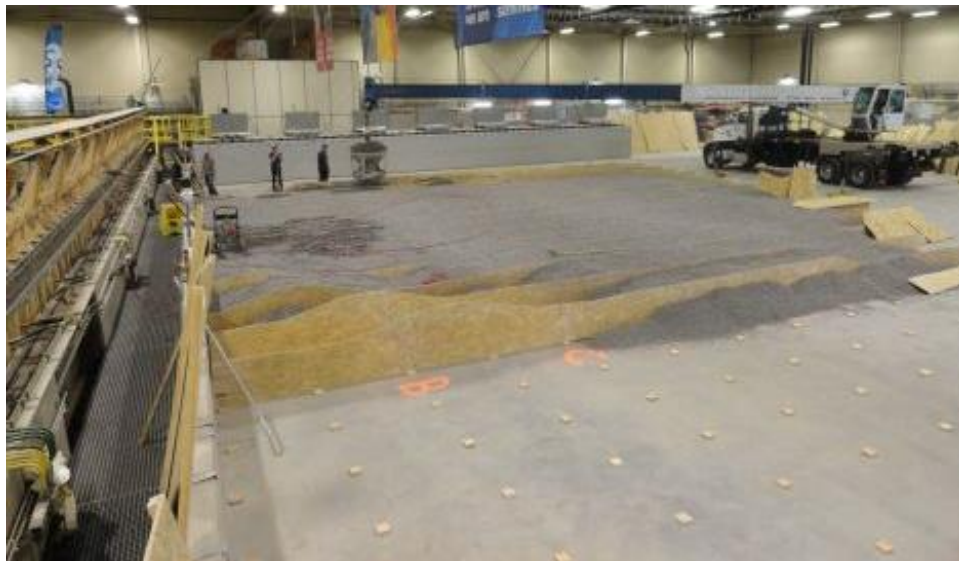
Figure 28. Heavy construction equipment was used to fill templates.
