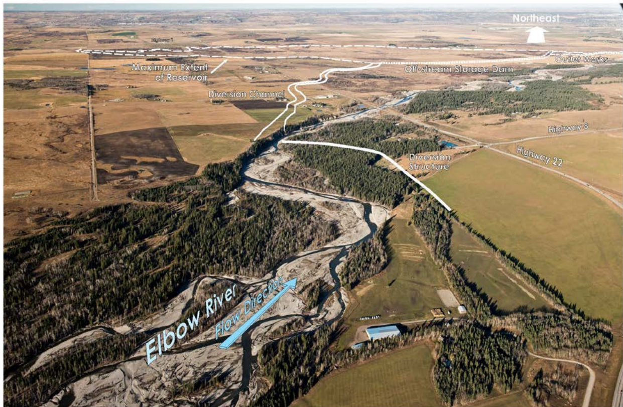
Figure 3-4 Looking Northeast towards Diversion Structure, Diversion Channel, Off-stream Storage Reservoir and Off-stream Storage Dam Locations
