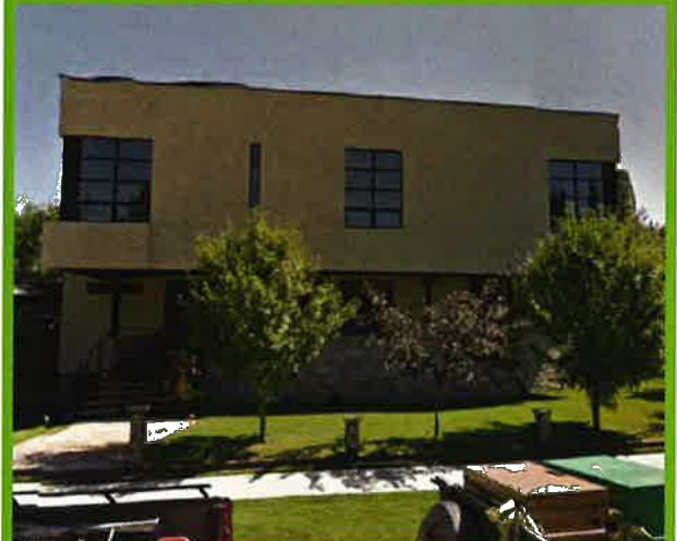
Elevated main floor with wall
