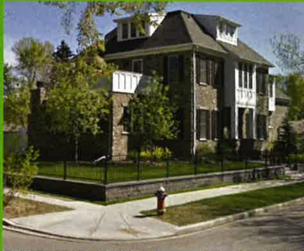
Elevated Lot and main floor with no basement
