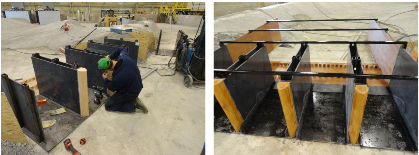
Figure 39. Left: installing the pier noses. Right: installing the support struts, rear retaining walls and rear stilling basin chute blocks.
