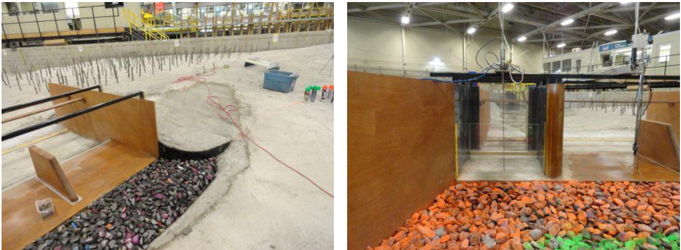
Figure 44. Left: the riprap apron was installed, and the (black) curved retaining wall on the RHS of the service spillway was tapered to match the profile of the floodplain berm. Right: view of the finished sluiceway with the clear plastic gate lowered and riprap painted orange.
