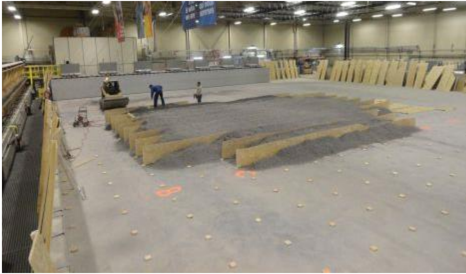
Figure 27. Fibreglass templates were erected and backfilled with fine gravel.
