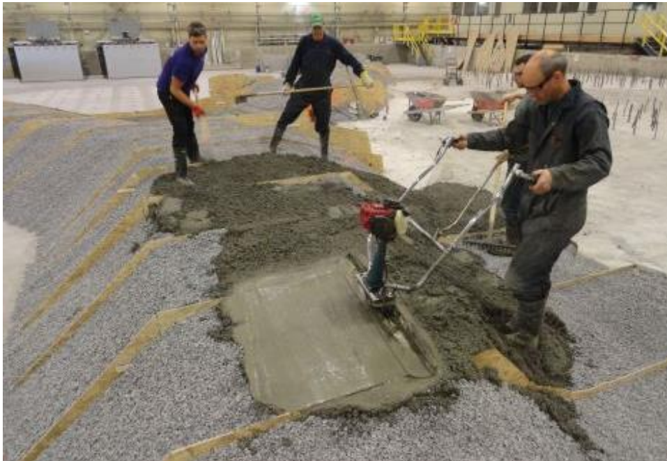
Figure 30. The concrete was screeded to match the template surfaces.
