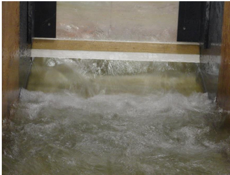
Figure 86. Unobstructed flow passing under the sluiceway gate ( 320 \text{ m}^3/\text{s} ).
