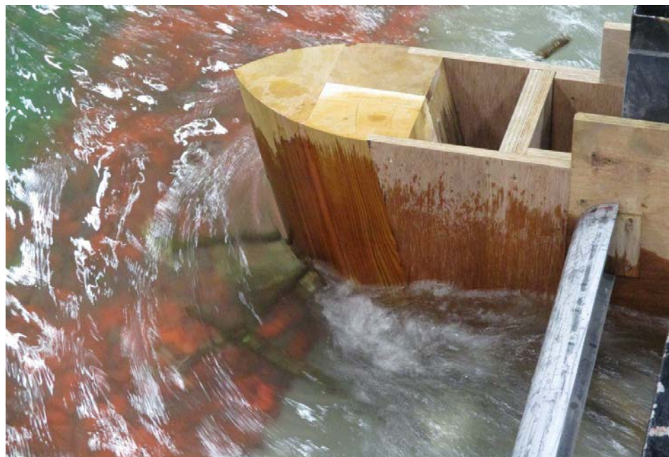
Figure 145. Debris caught on Pier Nose 3.
