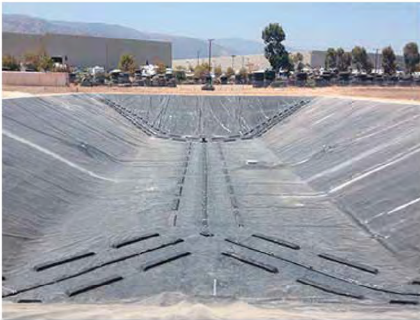
Figure 25. Reclaimed water storage reservoir floating cover fabricated with Enviro Liner® 6060, Corona California
