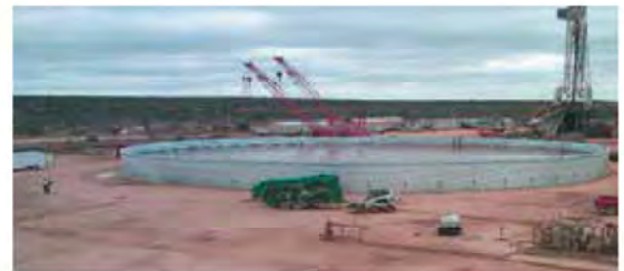
Figure 20. Enviro Liner® 6030 Frac Tank Liner, West Texas.
