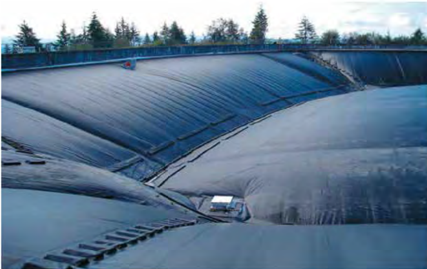
Figure 28. Floating cover being inflated during inspection
