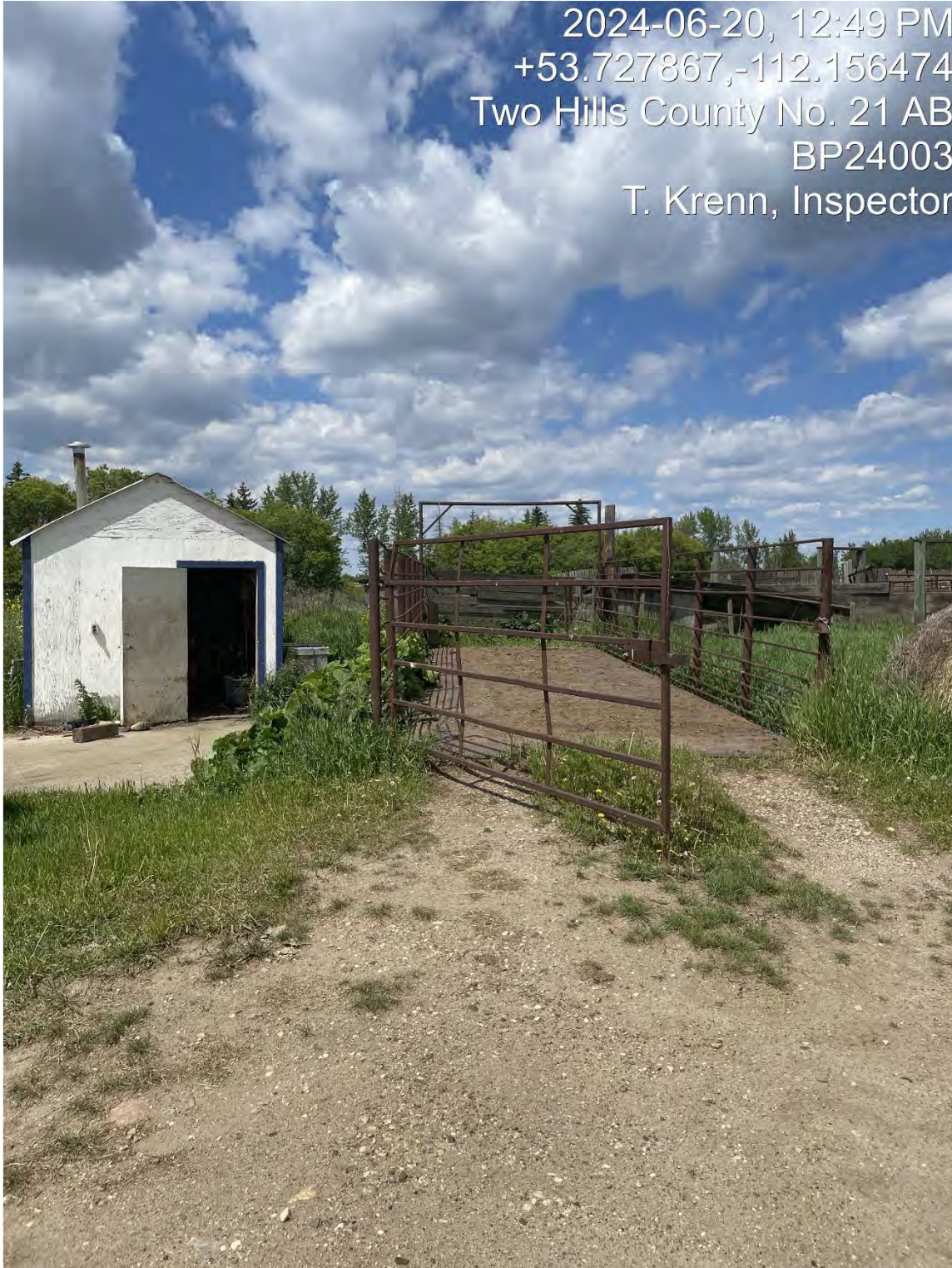
Looking northwest from the southeast side of the pumphouse and scale
