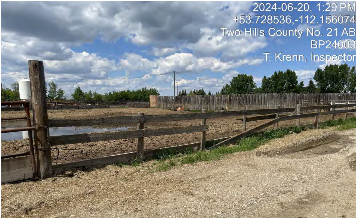
Pen 2 – looking west/northwest from the east fenceline
