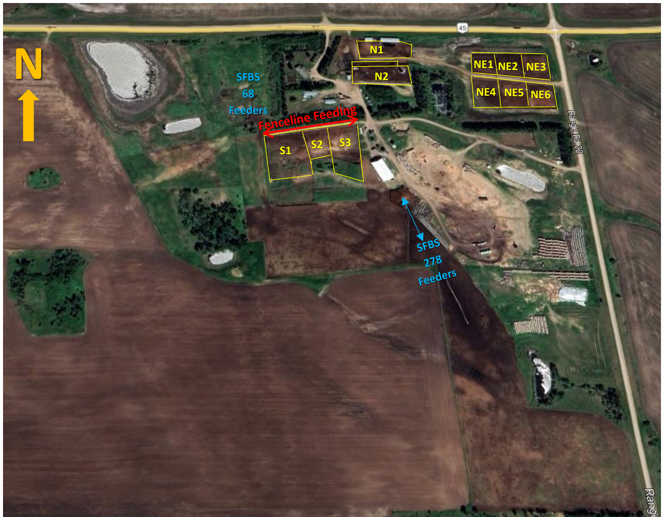
Site Inspection: January 29, 2025. Labelled by T. Krenn, Inspector
